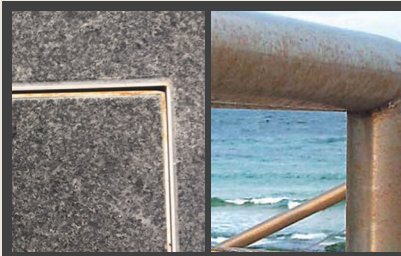
Photo showing 'Tea Staining' on Stainless Steel.
